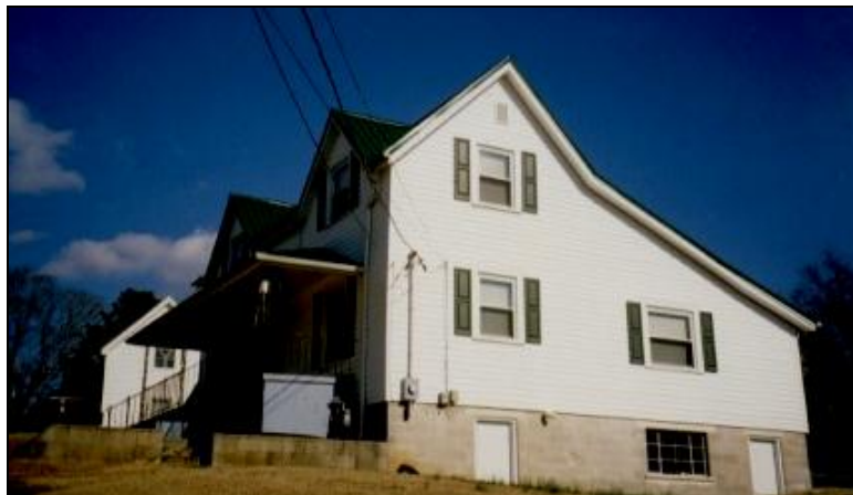
Figure 7.2 Early Two Story House, Piedmont, South Carolina.
