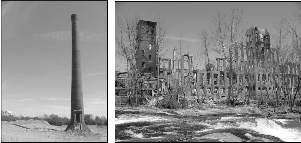
Figure 6.4 Site of the razed Spartan Mills (left) and Glendale Mill after the fire, March 27, 2004 (right)
