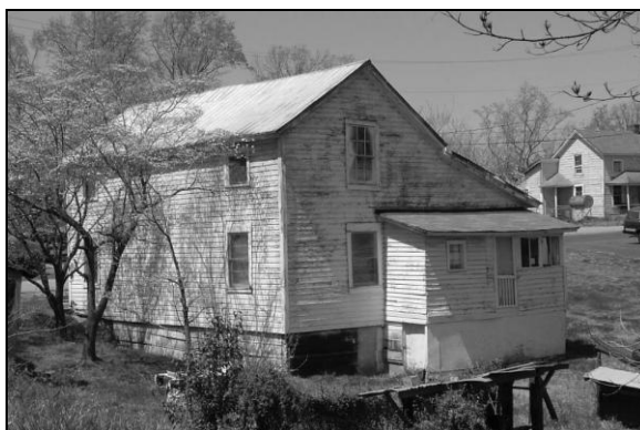
Figure 6.6 Deteriorated housing, Converse, Spartanburg County. March 2004
