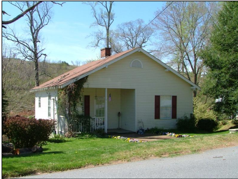
Figure 4.3 Front gabled cottage, Fingerville, Spartanburg County, SC, 2004
