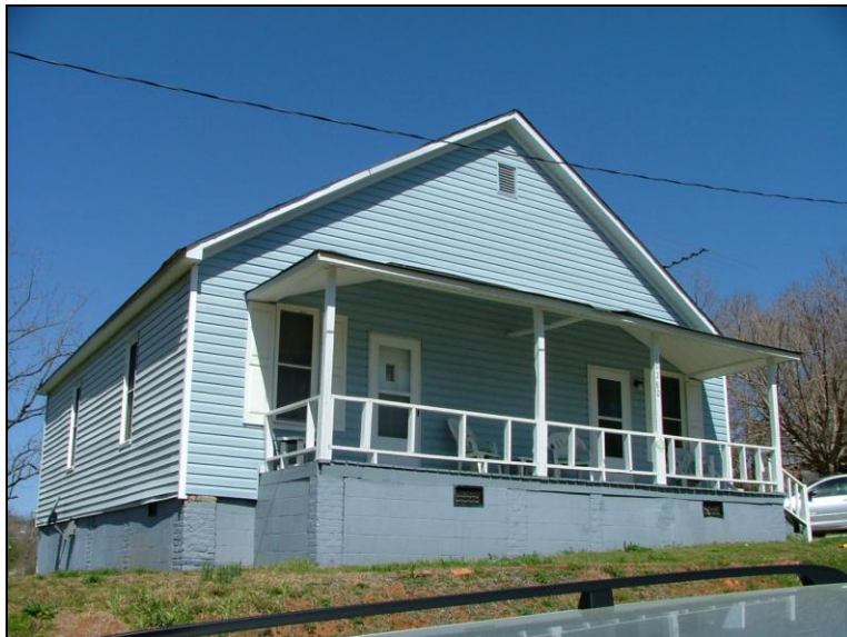
Figure 4.4 Front gabled duplex cottage, Fingerville, Spartanburg County, SC, 2004
