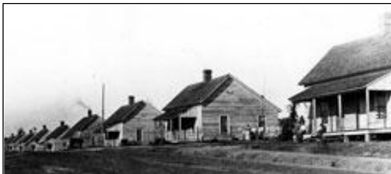
Figure 4.1 Saltboxes in Graniteville Source: Carolinana Library
