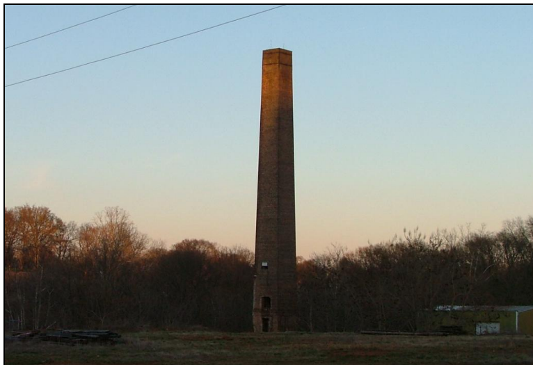
Figure 7.14 Smokestack, Piedmont, Anderson County, 2004.
